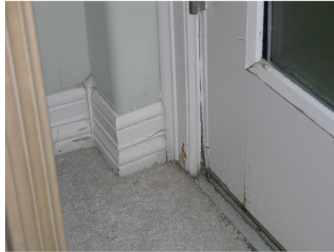
Figure 27.1 - Door leakage
