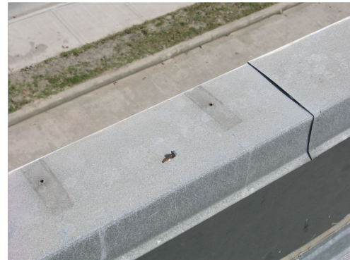
Figure 27.3 - Cap flashing openings
