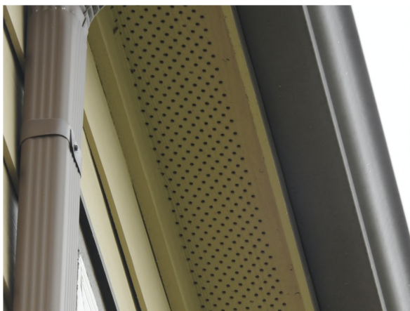
Figure 25.1 - Soffit vents
