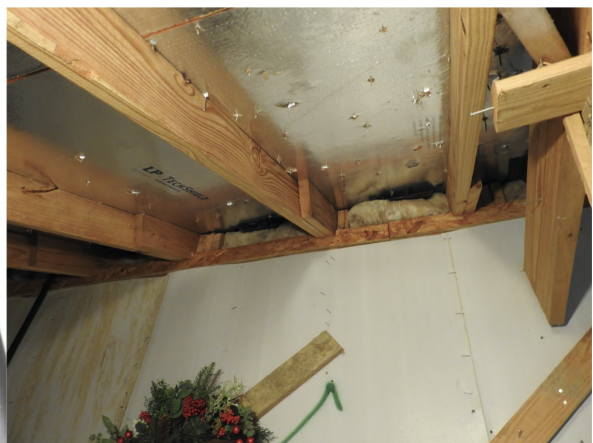
Figure 25.2 - Compressed rafter vents
