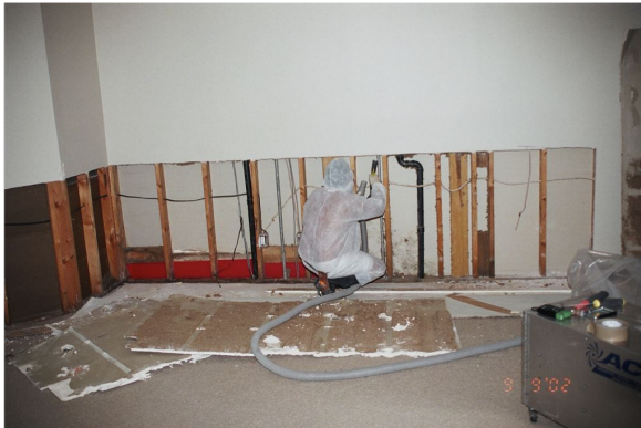
Figure 23.1 - Mold decontamination
