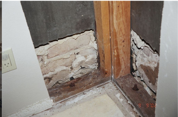
Figure 23.2 - Sheathing removed
